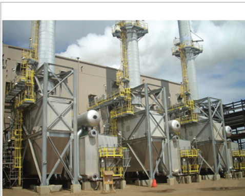
4. New packaged boiler design. Cleaver-Brooks has designed a high-efficiency, low-NO x elevated drum package boiler that generates 426,000 lb/h of steam at 550 psig and that minimizes field erection time. Courtesy: Cleaver-Brooks Engineered Boiler Division
