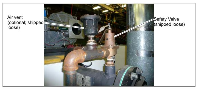
Figure 1-9 Boiler safety valve & air vent
