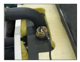
Figure 1-11 Outlet Temperature Sensor, Top of Pressure Vessel
