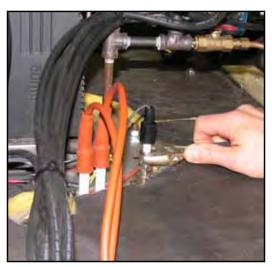
Figure 5-4 Tightening Flame Rod
