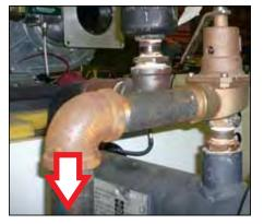
Figure 2-25 Pressure relief valve piped to safe point of discharge
