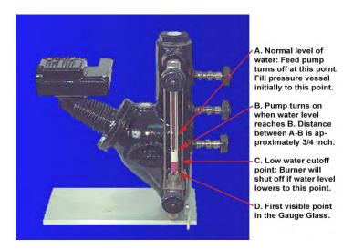
FIGURE 2-3. Boiler Water Level Details (Steam Boiler)
