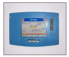
Figure 4-4 CB Falcon Display/ Operator Interface
