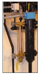
Figure 5-3 Water column gauge glass
