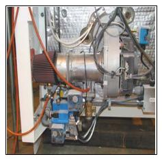
Figure 4-11 Blower Housing, Gas Valve & Mixing Venturi
