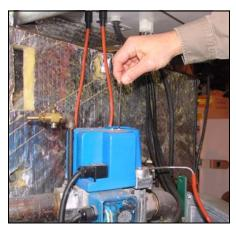
Figure 4-19 Main Gas Choke -High Fire Adjustment
