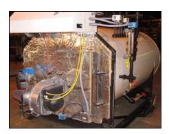
Figure 5-4 Front burner access panel removed
