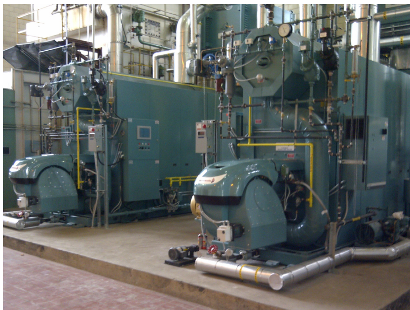
Cleaver-Brooks Large FLX gets up to steam quickly and can obtain 81 percent efficiency on steam applications and 85 percent efficiency on hydronic applications.
