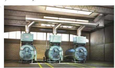
Stack designs for condensing boilers differ from those for near-condensing boilers.
