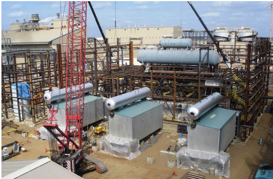
Fig 4: (Addendum) Elevated Drum package boilers, each rated for 426,000 lb/hr, shown during installation. A total of five(5) units were supplied on this project for a major oil producer.
