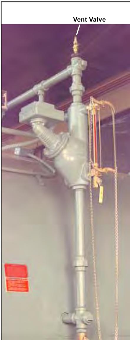
**Figure 2-11. Vent Valve on Water Column**
