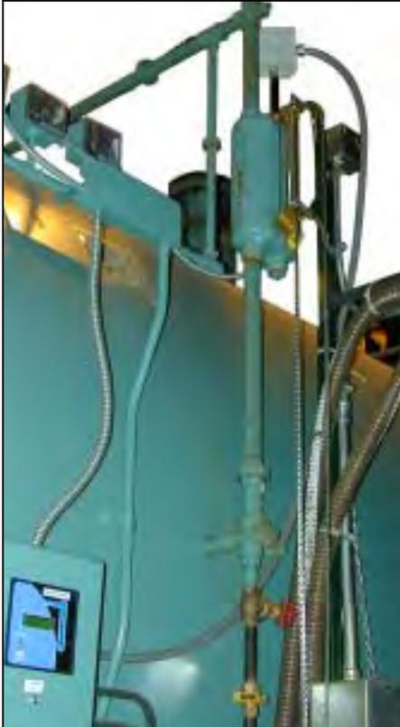
**Figure 2-1. Water Column with Level Master**
