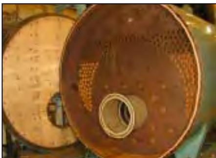
**Figure 1-3 Criterion 4WG Rear Access Way with Rear Door Open**
