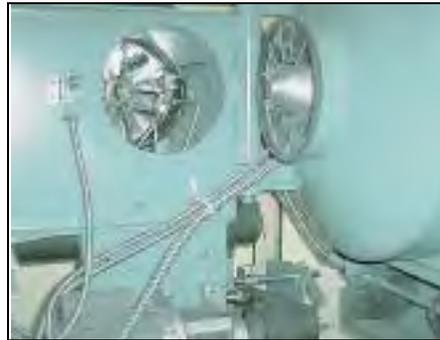
Figure 5-11 Burner Swung Out for Service
