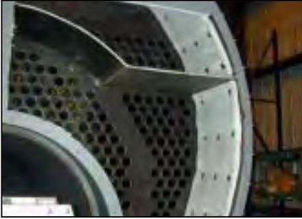
**Figure 1-6 Front Baffle
