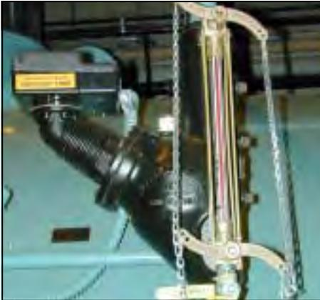
Figure 2-5. Low Water Cut Off
