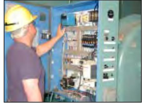
Figure 5-3 Flame Safety Inside Burner Control Panel
