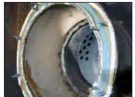
**Figure 1-5 Access Way to Second Pass Turnaround Chamber**
