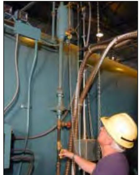
**Figure 2-10. Blowing Down the Water Column**
