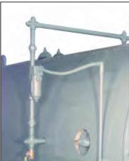
**Figure 1-11 Auxiliary Low Water Cutoff**
