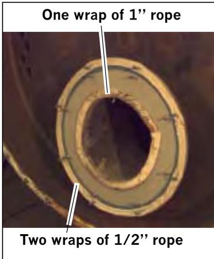
**Figure 2-14 Rope Gasket on Rear Access Way**
