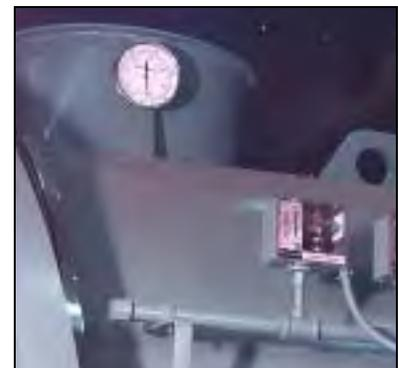
**Figure 2-7 Stack Thermometer**
