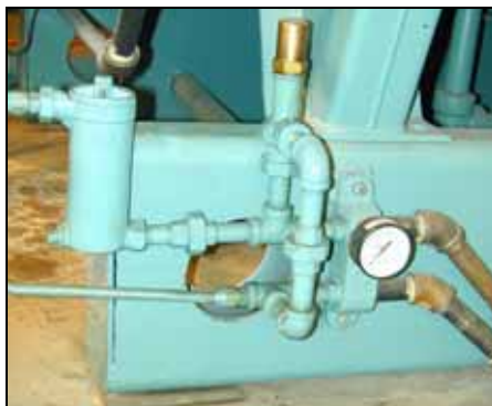
Figure 2-18 Terminal Block and Relief Valve
