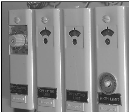
Figure 1-9 Hot Water Controls
