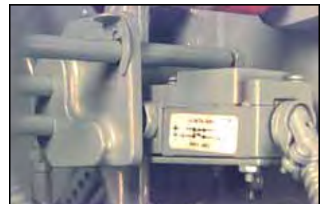
Figure 2-15 Oil Drawer Switch
