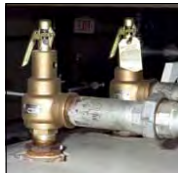
Figure 1-10 Safety Valves
