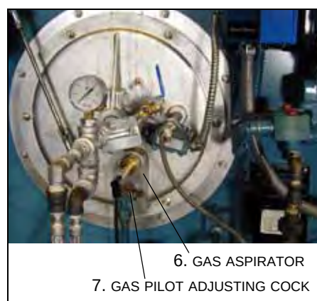
Figure 2-12 Burner Drawer Face
