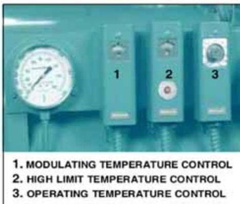
FIGURE 1-5. Temperature Gauge and Hot Water Controls
