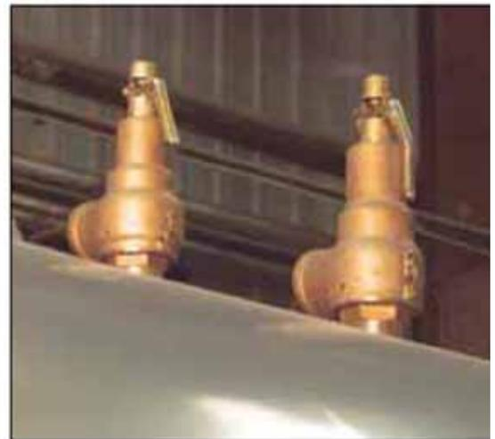
FIGURE 1-4. Safety Valve Piping and Safety Valves
