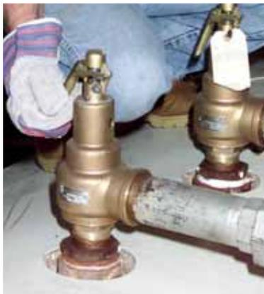
Avoid excessive operation of the safety valve; even one opening can provide a means of leakage. Safety valves should be operated only often enough to assure that they are in good working order. When a pop test is required, raise the operating pressure to the set pressure of the safety valve, allowing it to open and re-seat as it would in normal service.
