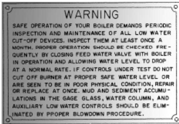
**FIGURE 8-3. Low Water Cutoff Plate**
