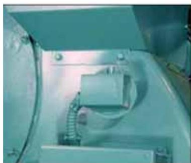
Air pressure against the diaphragm actuates the switch which, when made, completes a circuit to prove the presence of combustion air. since the pressure of the combustion air is at its minimum value when the damper is full open, the switch should be adjusted under that situation. It should be set slightly below the minimum pressure, but not too close to that point to cause nuisance shutdowns.
