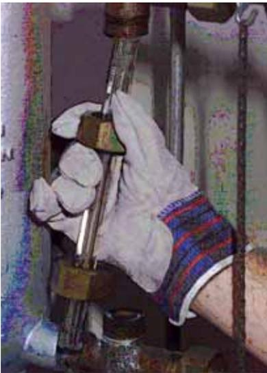
It is recommended that the boiler is off and cool when the glass is replaced.
