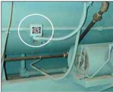
The air pressure against the diaphragm actuates the switch which, when closed, completes a circuit to prove the presence of atomizing air. Since the pressure of the atomizing air is at its minimum value when there is no fuel present at the nozzle, adjustment of the switch should be done while the unit is running but not firing. The control should be set slightly below the minimum pressure, but not too close to that point to cause nuisance shutdowns.
