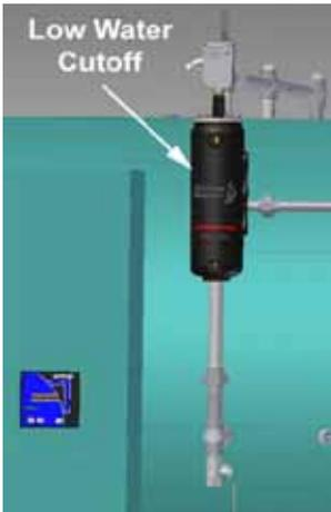
Always be sure of the boiler water level. On steam boilers, the water column should be blown down daily. Check samples of boiler water and condensate in accordance with procedures recommended by your local Cleaver-Brooks authorized representative. Refer to Chapter 3 for blowdown instructions.
