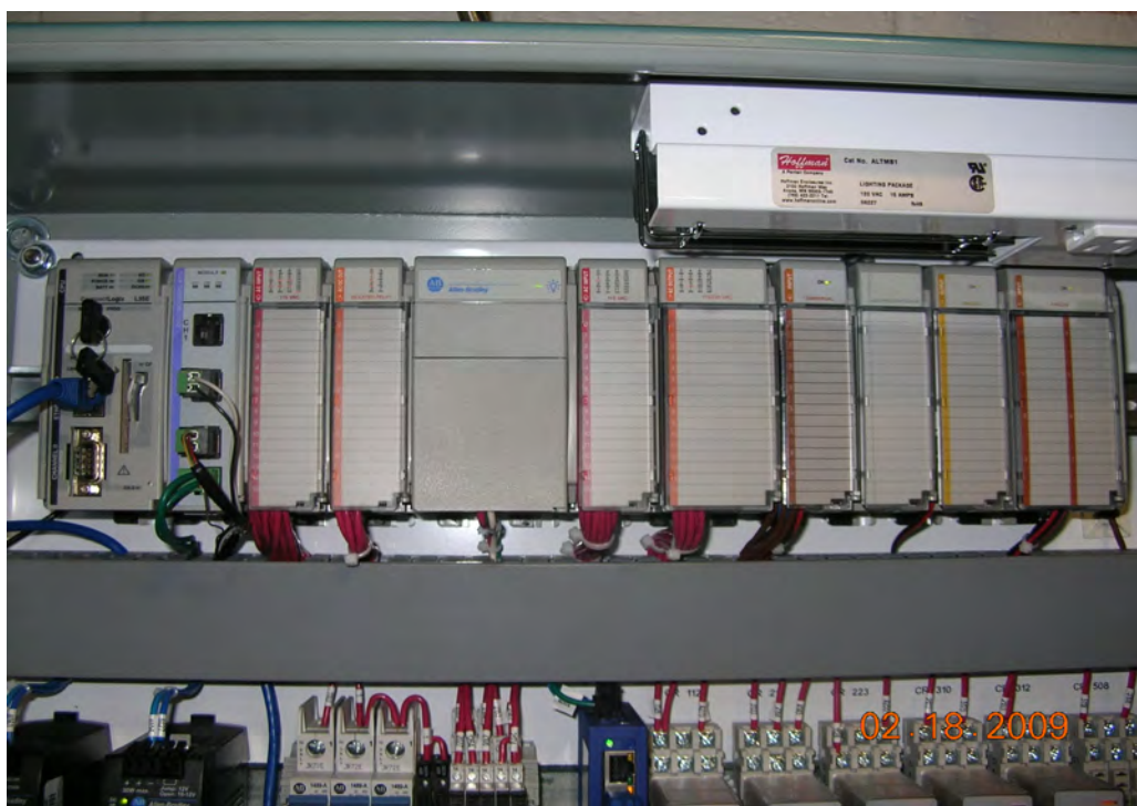
Figure 3-1 PLC Module Assembly
