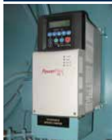
Variable speed drive
