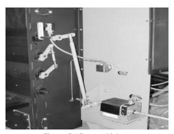
Figure: 5-6 Damper Linkage
