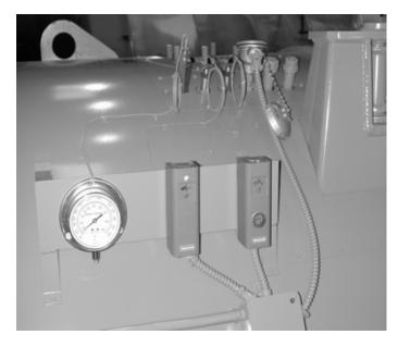
Figure 4-3: Hot Water Operating Controls
