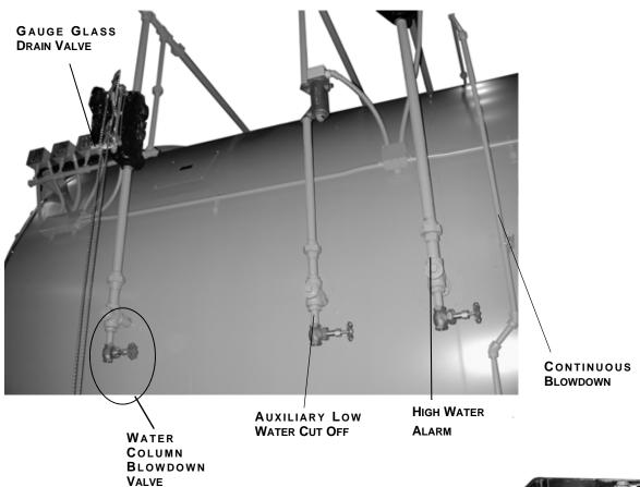
Figure 1-5: Water Column Assembly
