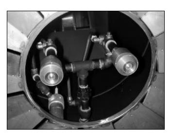
Figure: 5-5 Oil Nozzles and Pilot
