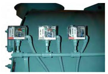
Figure 4-2: Steam Operating Controls
