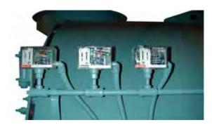
Figure 4-5: Steam Operating Controls
