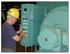
Figure 6-2. Burner Control Panel
