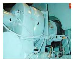
1. BLOWER MOTOR 2. COMBUSTION AIR PROVING SWITCH 3. BLOWER HOUSING
