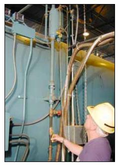
Figure 9-2. Low Water Cut Off Blow Down
