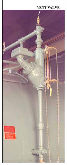
Figure 2-8. Vent Valve on Water Column
