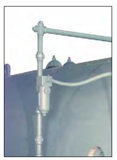
Figure 1-10. Auxiliary Low Water Cutoff
