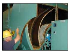
Figure 1-5. Front Baffle Four Pass Design
