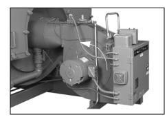
Figure 4-4. Fan Motor ICB ProFire
