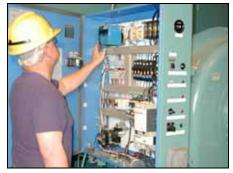
Figure 6-3. Flame Safety Inside Burner Control Panel
