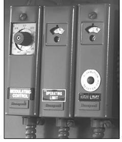
Figure 5-3. Hot Water Operating Controls
