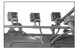
Figure 4-8. Pressure Controls
