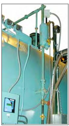
Figure 1-9. Water Column and Low Water Cut-Off
