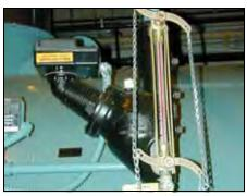
Figure 9-4. Low Water Cutoff Gauge Glass
