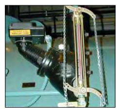
Figure 2-5. Low Water Cut Off
