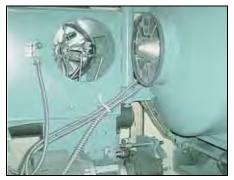
Figure 6-9. Burner Swung Out for Service
