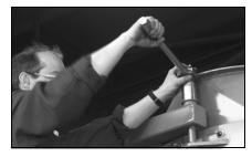
Figure 9-12. Release Tension on Davit Arm After the Door is Secured in Place
