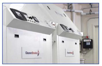
Cleaver-Brooks hydronic controls combinine PID set point and outdoor reset algorithms, boiler sequencing and firing rates, and pump speed controls into one control system for more efficient boiler operation.
