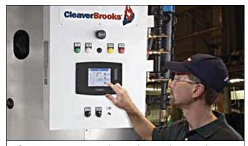
**The FALCON** – is an advanced control system for optimum boiler control for individual and multiple units on both the steam and hot water ClearFire boilers.
