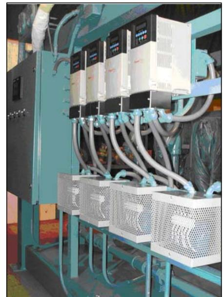
**Figure 2-12 Variable Frequency Drives**
